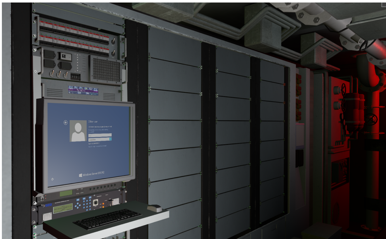
Figure 2-2: Interactive Line Replaceable Units can be viewed within a 3D virtual environment, as they would be seen within the compartment on the operational platform.
